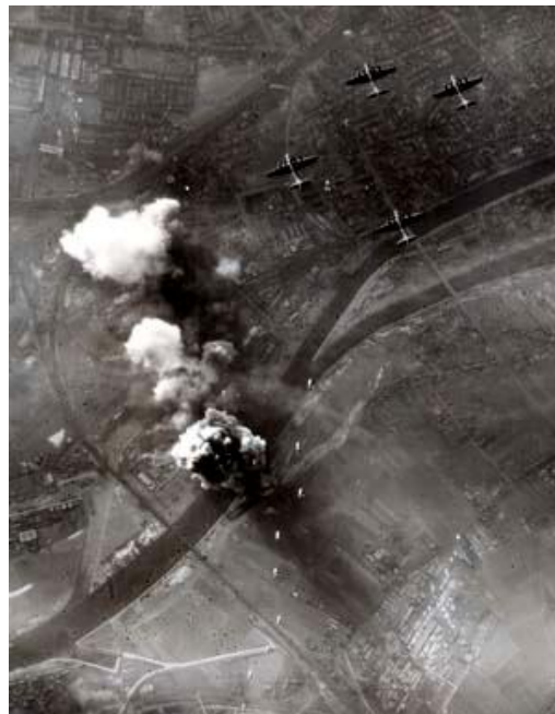
15 th Air Force bombers score hits on oil storage facilities in Regensburg, Germany.
