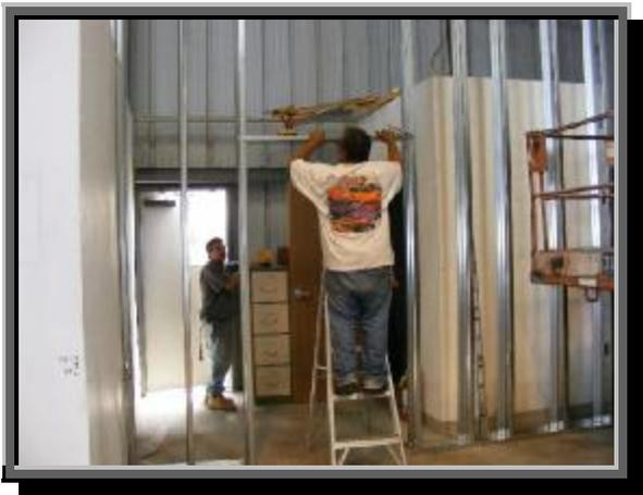
**Workmen installing framing for one of the doors in the new firewall. The men's and women's rooms were left intact, with the framing forming a separate wall on the west side of them.**
