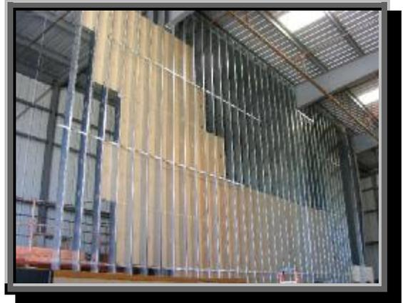
**Insulation being installed before the dry-wall goes on the maintenance hangar side of the wall.**
