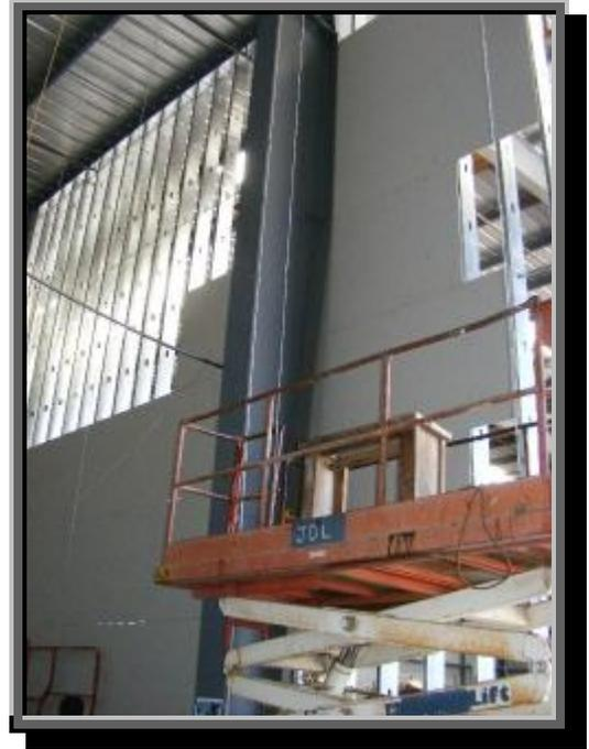
**This shot, taken between the outside wall and the new wall, shows the existing girder and the dry-wall being installed.**
