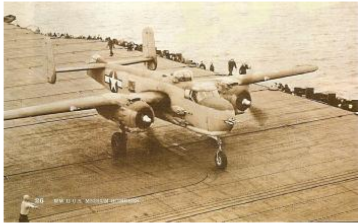
© Photo courtesy WWII Medium Bombers, Fall, 2006 A USMC PBJ-1H (3-toned, grey & blue) Mitchell bomber going through sea trials on USS Shangri-La (CV-38), an Essex-class carrier, on November 15, 1944 off Norfolk, VA. This PBJ, heavier than the Doolittle B-25Bs, made an arrested landing on the Shangri-La.
