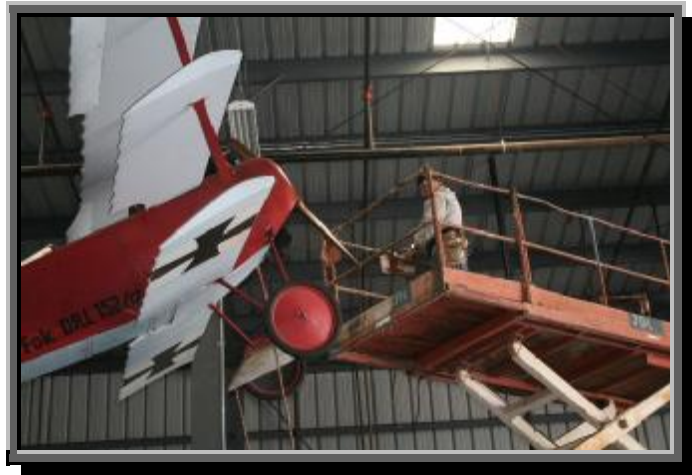
© Photo by Ron Fleishman Jim Hinkelman and Jake Lombard up on the scissor-lift attaching the hanging bridle to a steel wire rope.
