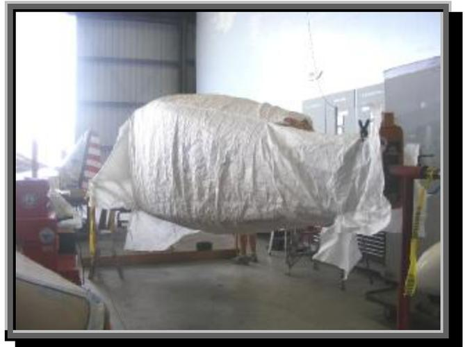
View from the tail. The fabric will tighten to the fuselage as it is heated. No stitching will be necessary, as was the case with the wings. George, Barry, and Mike Hohls & Norm Swagler will do the work soon.
