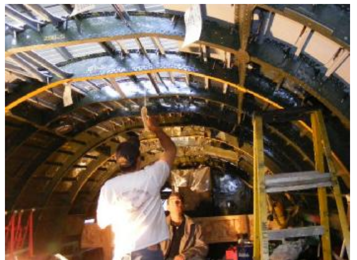
© Photo courtesy of Dan Newcomb Dan Newcomb and Scott Drosos riveting new panels.
