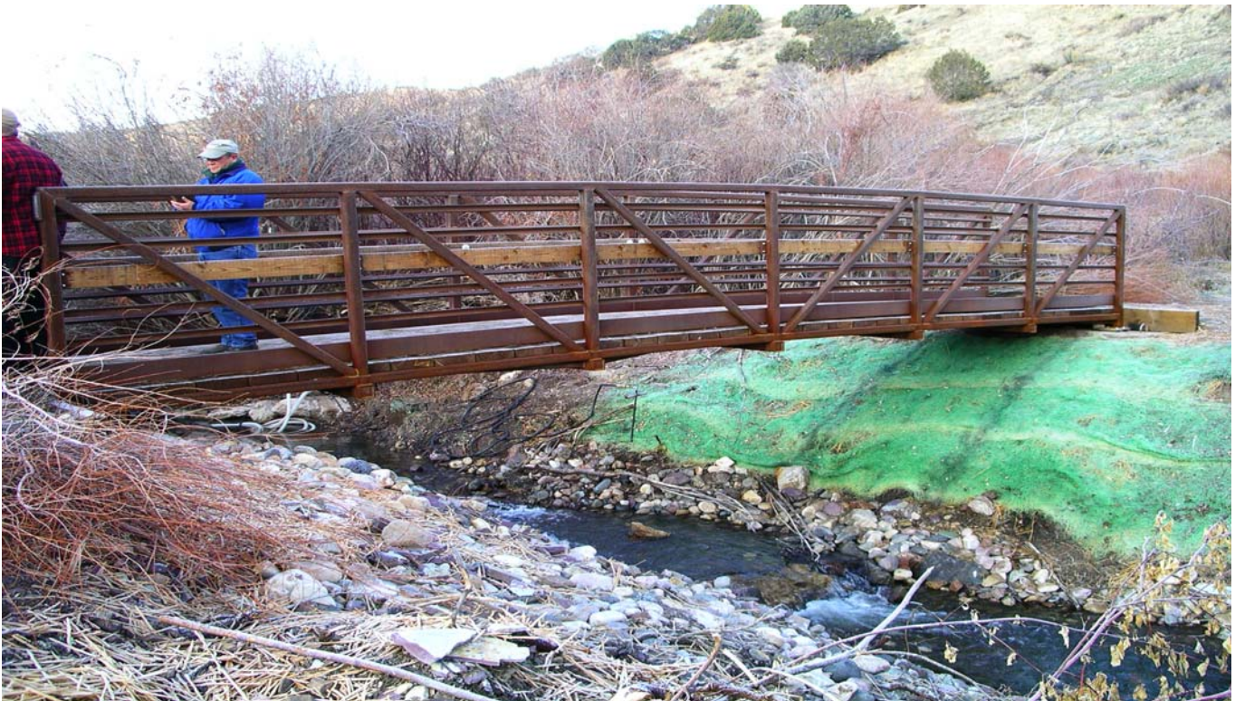
With a new foot bridge installed, the parking lot was moved to the highway side and the concrete culverts in the creek were removed and the area completely terraced with rock and erosion screens.
