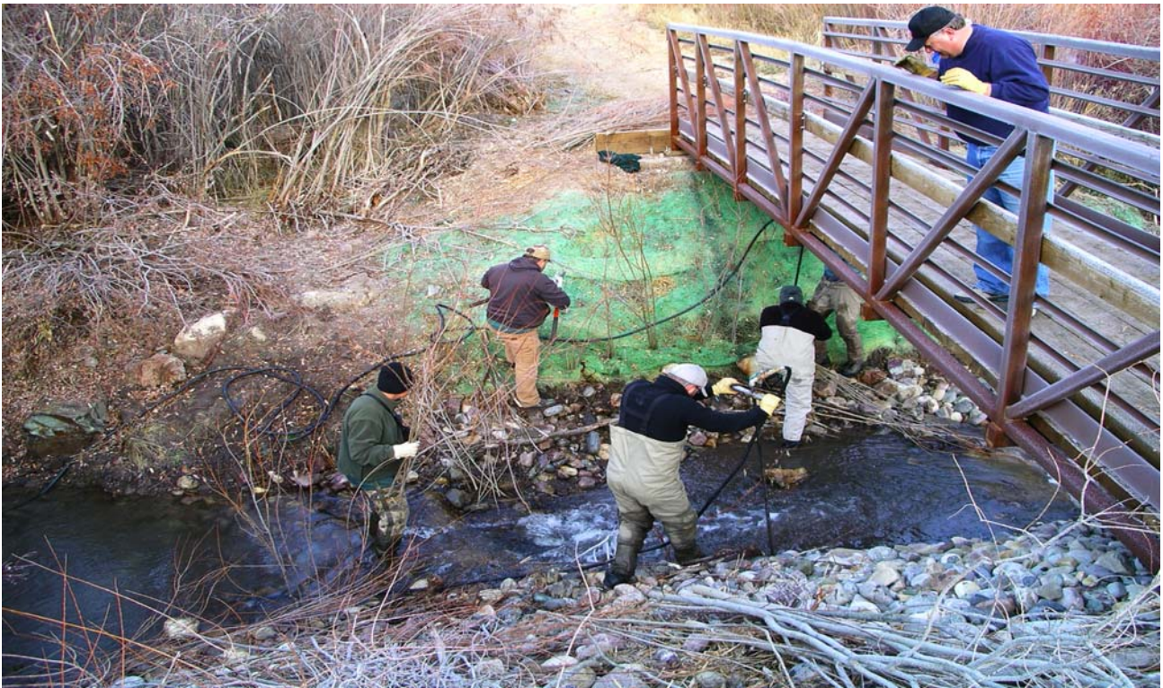
The stingers would bore holes into the bank and other volunteers were ready to insert a bundle of willow branches into the bored holes. Spring showers from the stingers were sometimes unavoidable!!
